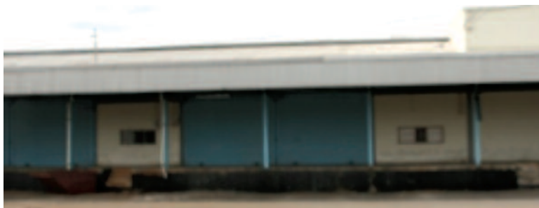
Figure 1: Model packing house built using concrete
