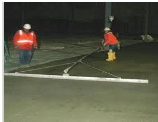
Figure 2: Steel floated floor surface
